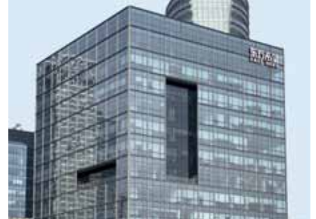
Helbling Representative Office, Shanghai, China
