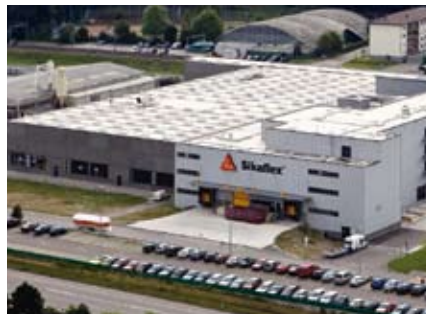
SIKA, Düringen: project controlling for construction of new production facility
