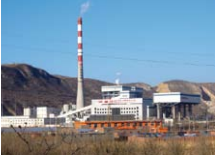
Thermal power plant in Nanzhuang, China
